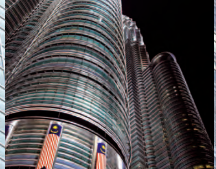
PETRONAS TOWERS | KUALA LUMPUR Pelli Clarke Pelli Architects
