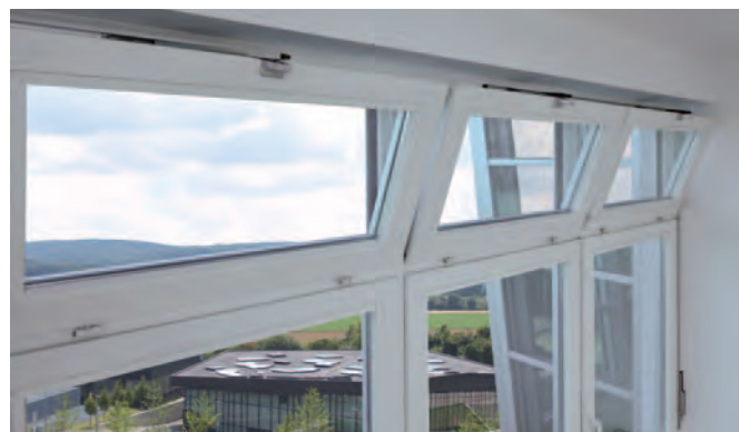
Manual or motor-driven operation for ventilation purposes
