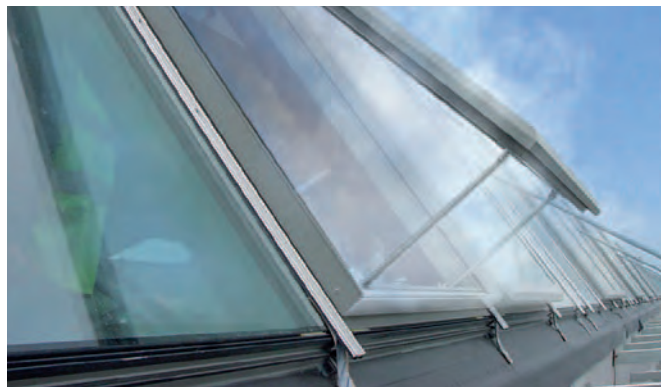
Low smoke density rescue routes with SHEV system solutions from GU
