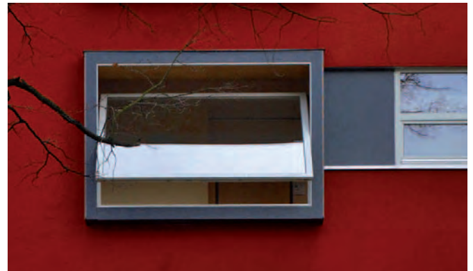
Horizontal-pivot window for sash weights up to 300 kg
