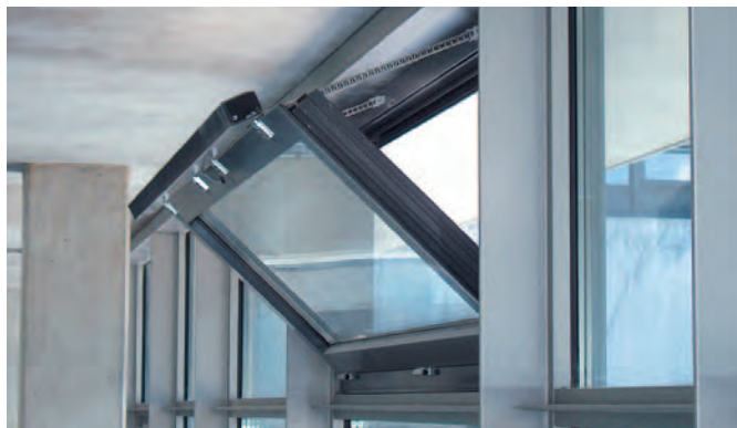
Chain drives ensure rooms receive the perfect amount of ventilation with opening widths up to 750 mm
