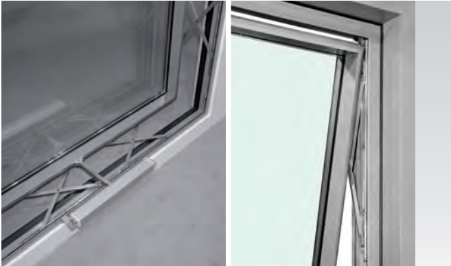
Sophisticated facade solutions using standard hardware
