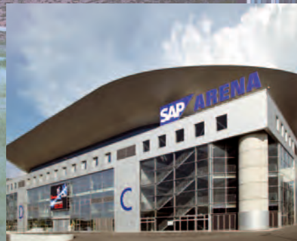
SAP ARENA | MANNHEIM Architects: HPP Hentrich, Petschnigg & Partner
